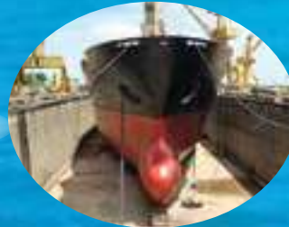
Ship Repair & Renovation
